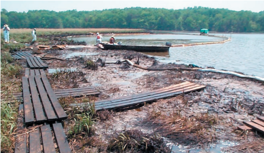
Removing oil from a wetland contaminated with heavy fuel oil—planking is used to reduce trampling.
