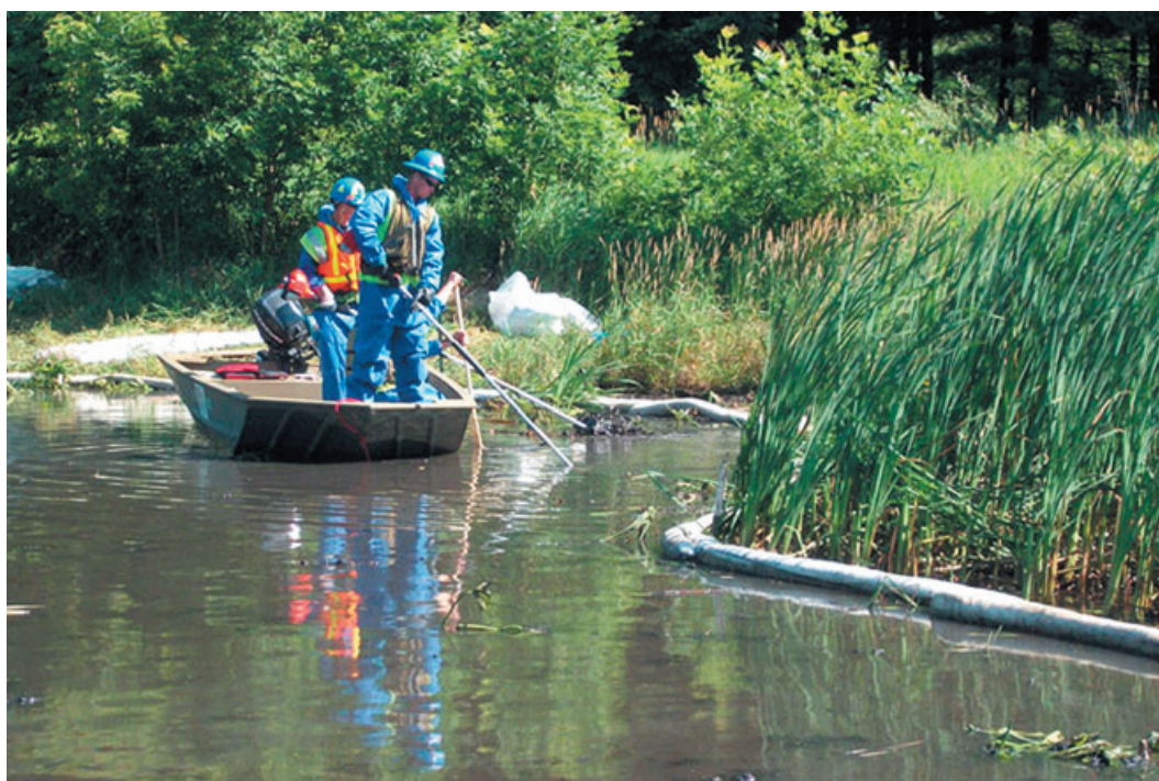
Pumping water into river sediment to release sunken oil and flush it to the surface.
